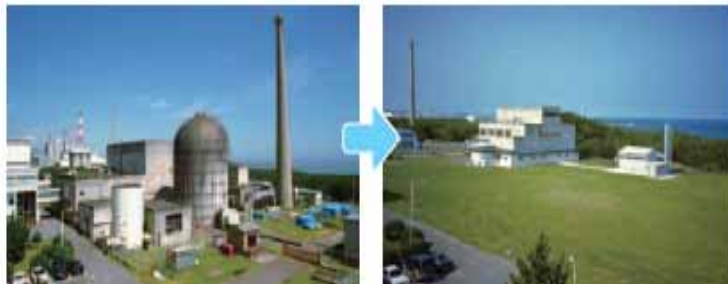
Decommissioning of the Japan Power Demonstration Reactor (of former Japan Atomic Energy Research Institute)
